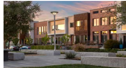
Park Moderns - 32 Single Family Homes (Completed) These 32 single-family homes surround Garden Park to create the sense of an outdoor room. Development was designed with California Urban Core living in mind.
