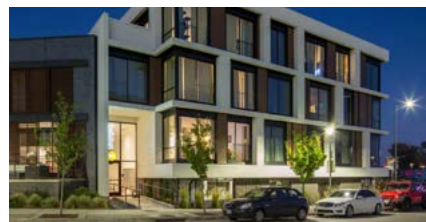
Habitat Apartments - 96 Units (Underway) The Habitat Apartments frame the four corners of Garden Park and are just steps away from a 1-mile long stretch of West Sacramento's Riverwalk.
